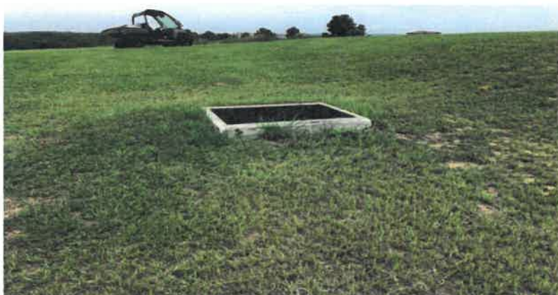
Pond #6 - Overflow Structure
