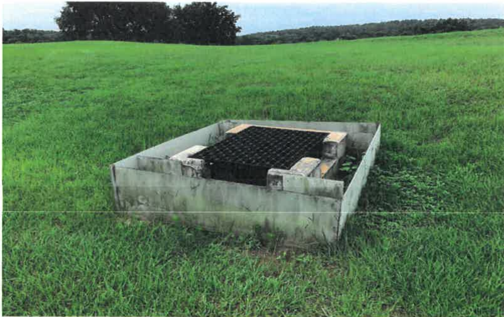
Pond #23 - Overflow Structure
